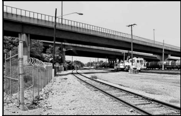
Mt. Clare Yard, under I-95 looking north where the proposed alignment would diverge to the left to meet the Hanover Subdivision.
