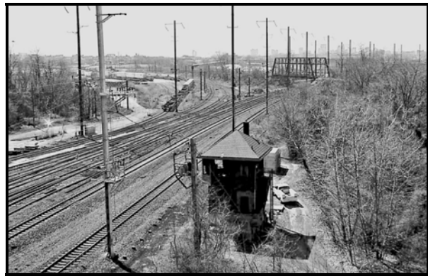
Looking west to the CSXT Railroad Bridge.
