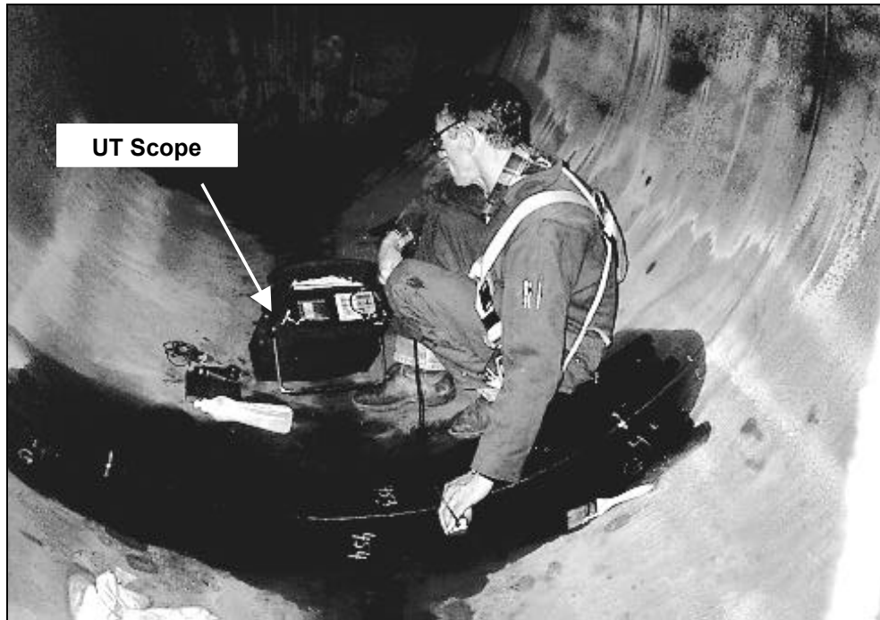
Figure 38. Ultrasonic Evaluation of the Transverse Butt Weld
