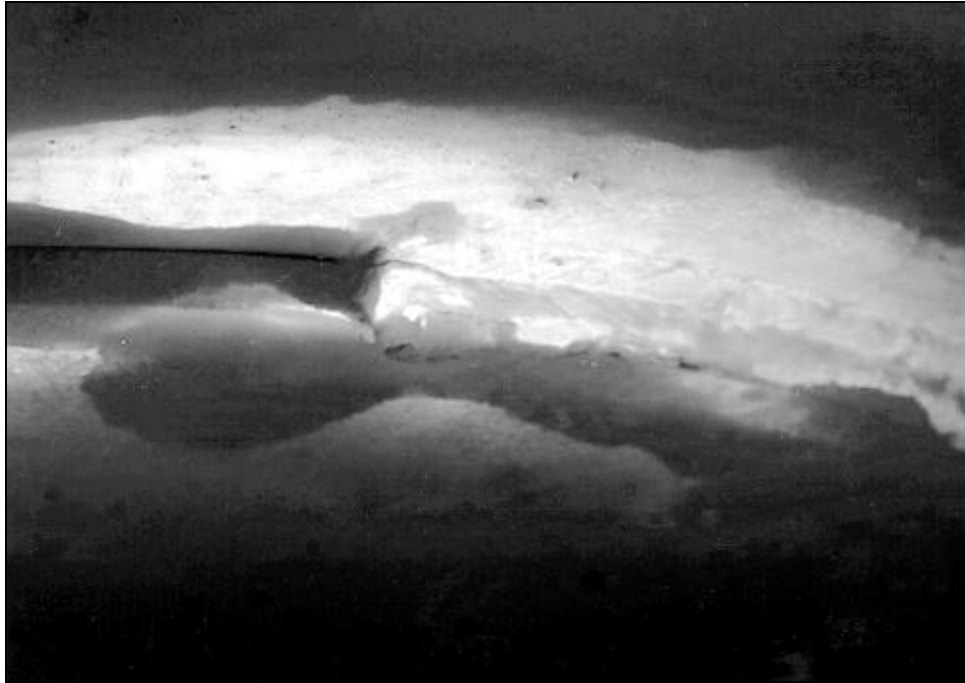
Figure 34. Liquid Penetrant Inspection Showing 0.050-inch Crack at Fillet Weld Termination of the Sill Bearing Plate
