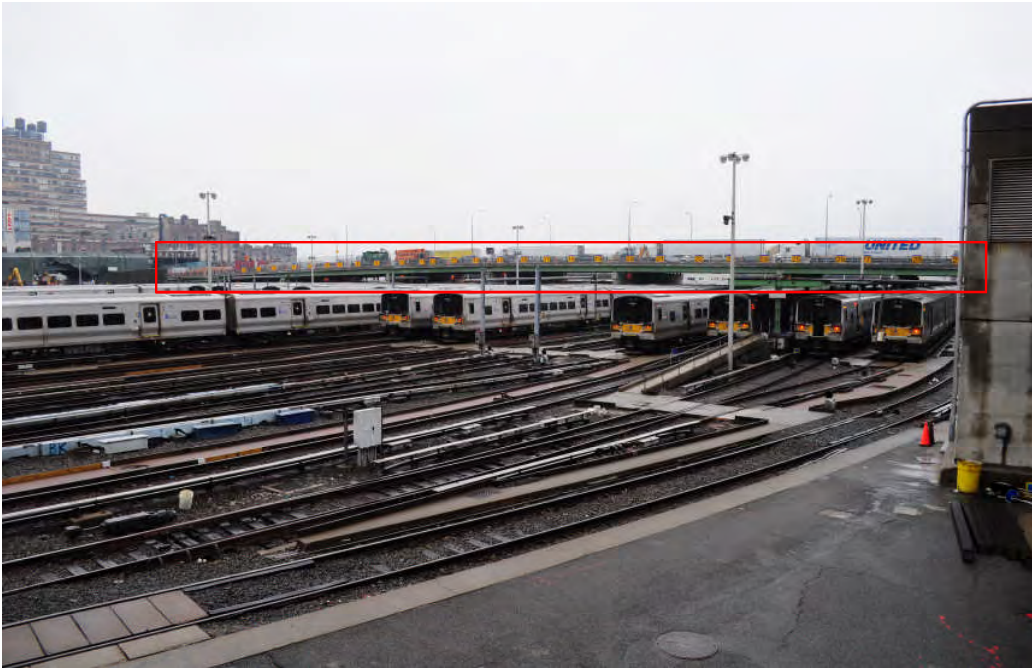
Eleventh Avenue Viaduct Looking South and West
