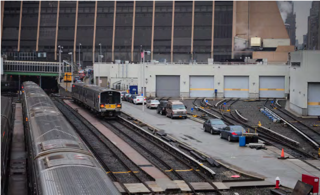
MOE Building Looking East from Eleventh Avenue Viaduct
