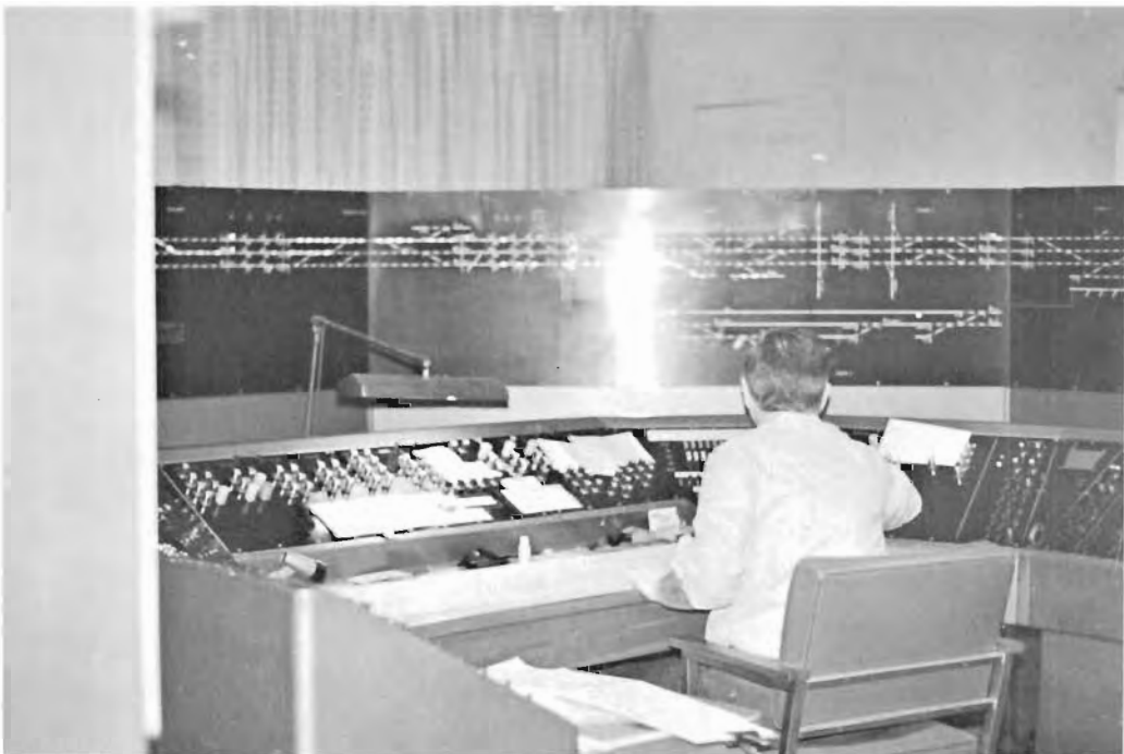
Figure 3-8. Separate CTC Board and Switching Console
