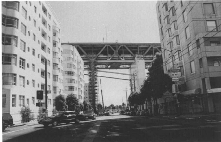
Fig 3B Main Street, Looking South to Bay Bridge Steel Work
