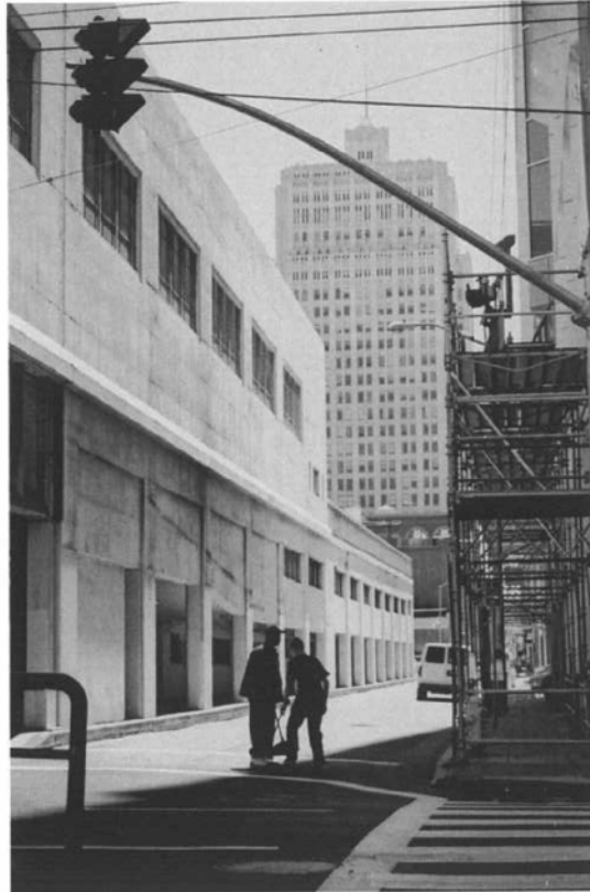
Fig 4A Pacific Telephone Building (New Montgomery Street) from Minna Street
