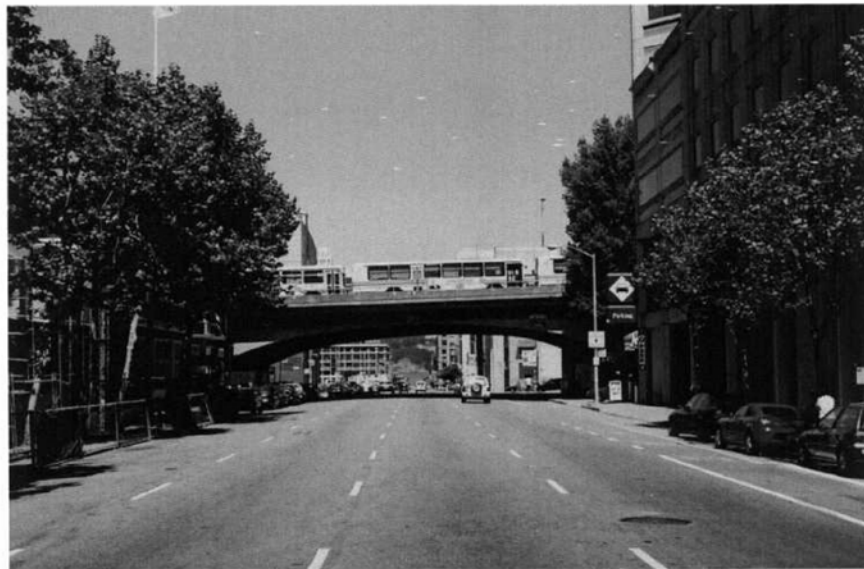
Fig 9B Folsom Street at Second Street, Looking East
