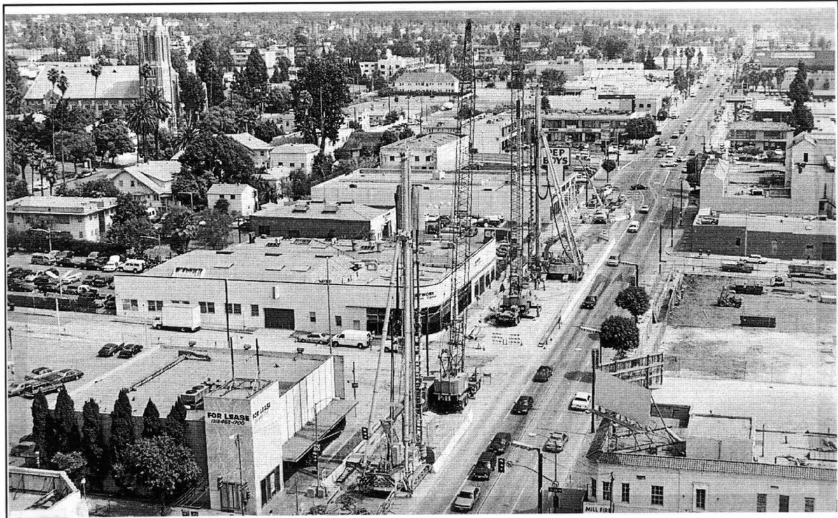
Figure 5.20-1: Soil Cement Wall Augers In Use
