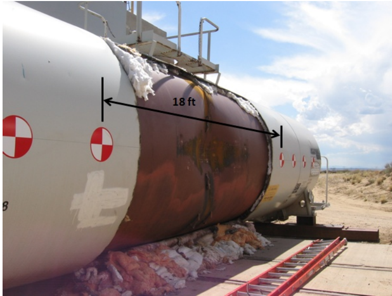
Figure 43. Deformation of Commodity Tank
