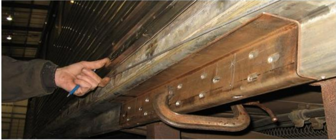
Figure 5. Steel Patch to Repair Fatigue Cracks
