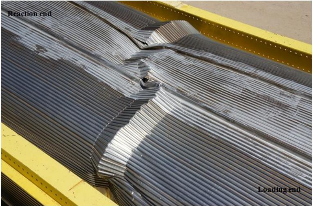
Figure 11. Crippling of Roof (Car 248)
