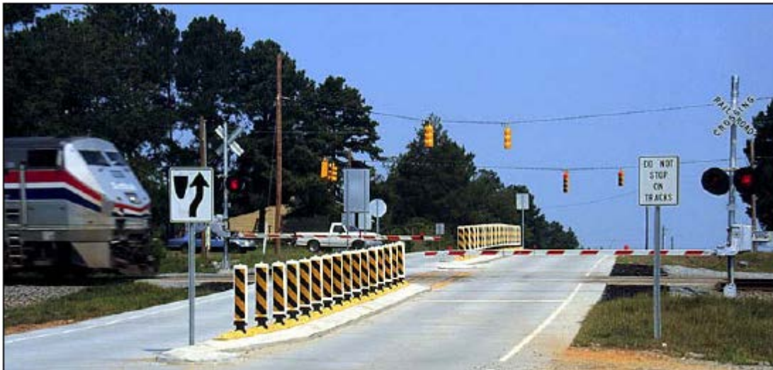
Figure 3.3. Traffic channelization device in North Carolina (FRA 2010)
