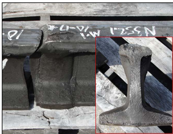
Figure 3. WGW O6 with Shelling on Gage Corner and Fatigue Fracture from Base of Weld—Inset Shows Fracture Face—Fatigue Initiated at Runout at Base of Weld
