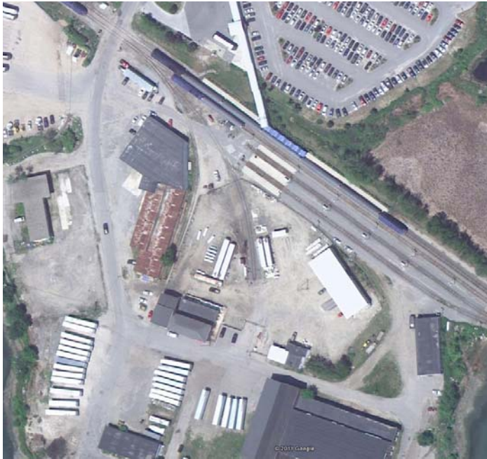
Photo 1: Portland Layover Facility
