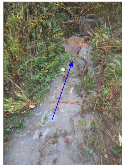
Site 2B Photos: Runoff from the unpaved lot and from nearby structure roofs drains to the stream (left). Sediment-laden water flows directly to the stream (right).
