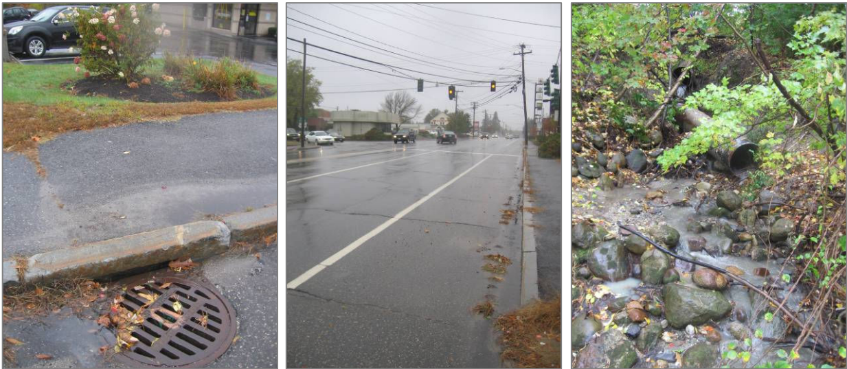
Site 1 Photos: Storm drain on Route 1 that is linked to the culverts behind McDonalds (left); view of area draining to the storm drain (middle); stacked culverts behind McDonalds (right).
