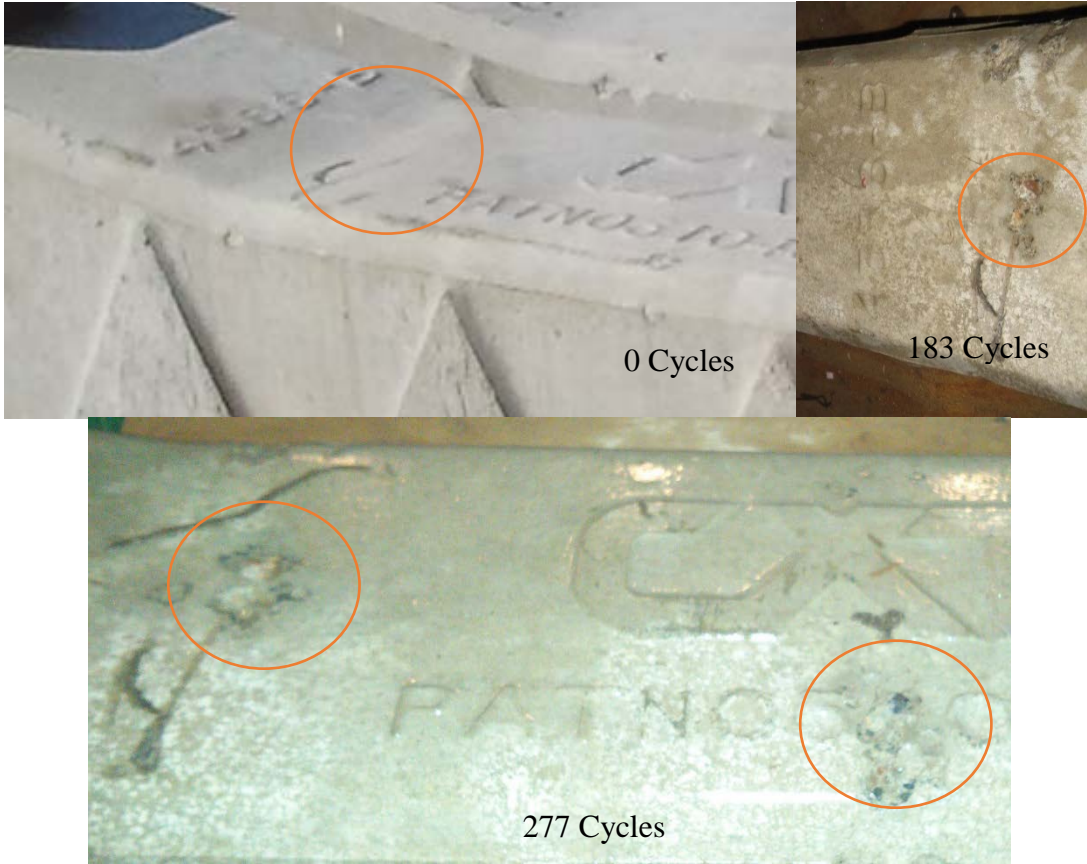
Figure 23: Tie #2-4386-B pop-outs and surface scaling.
