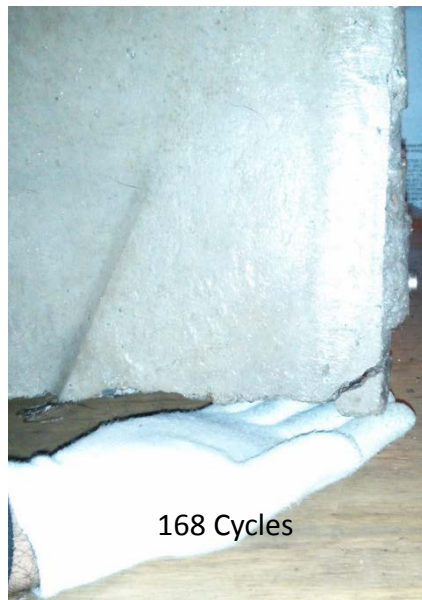
Figure 24: Tie #2-4386-B corner piece after fracture.
