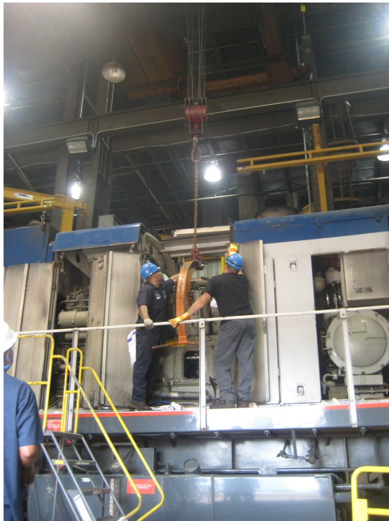
Figure 5: Amtrak personnel removing the 2R power assembly for inspection.
