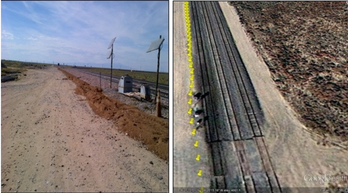
Figure 3: Side-by-Side Comparison of Installation Photo and GPS Survey Overlay
