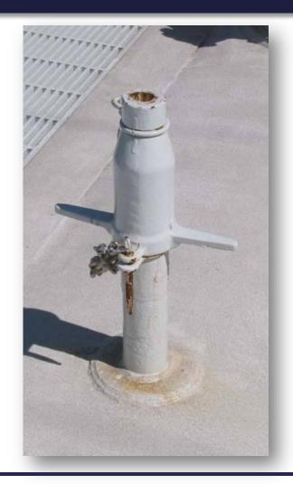
The bottom outlet plug and/or cap must remain off its fitting during entire loading process to ensure that the bottom outlet valve is not leaking.
