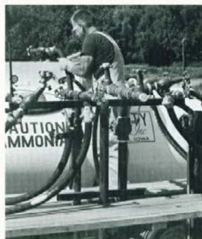
It takes nine minutes to fill a 1,000 gallon nurse tank at this bulk plant of Lavery Elevator, Inc., Indianola, Iowa. Two nurse tanks can be filled simultaneously at this dual load-out riser.
