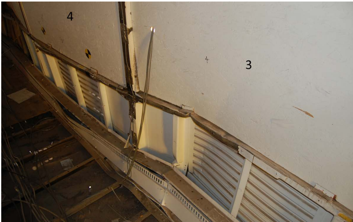
Figure 65. Damage to Left Side Interior of Car 244
