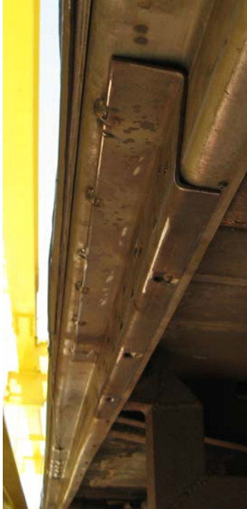
Figure 6. Patch Installed on Car 244 Side Sill
