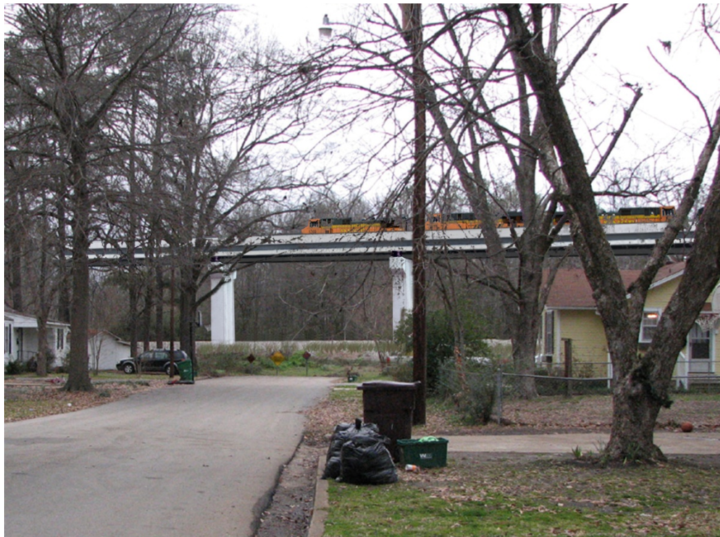
View Looking North within Gravlee District with Build Alternative
