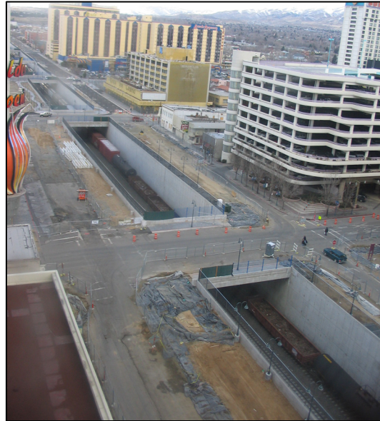
Railroad Trench in Reno, Nevada
