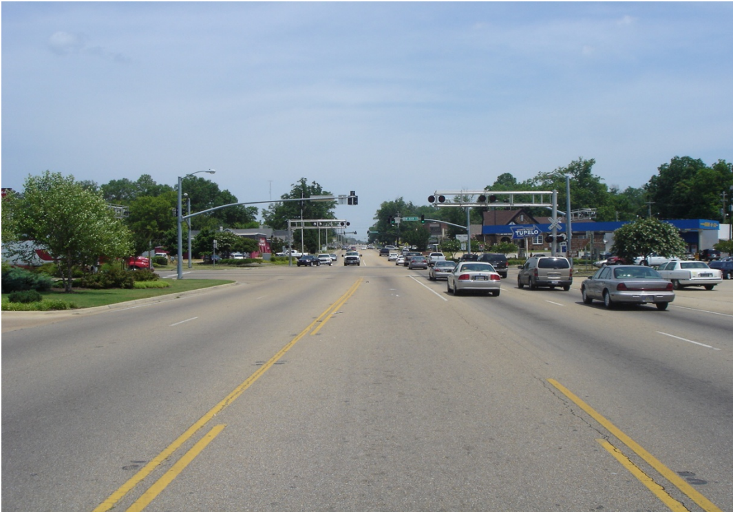
Existing View Looking North at Crosstown Intersection
