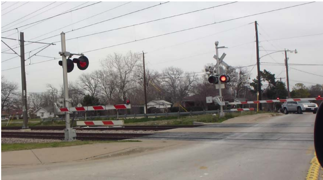
Figure 6. Gate Skirt Installation at Waco Ave., Dallas, TX
