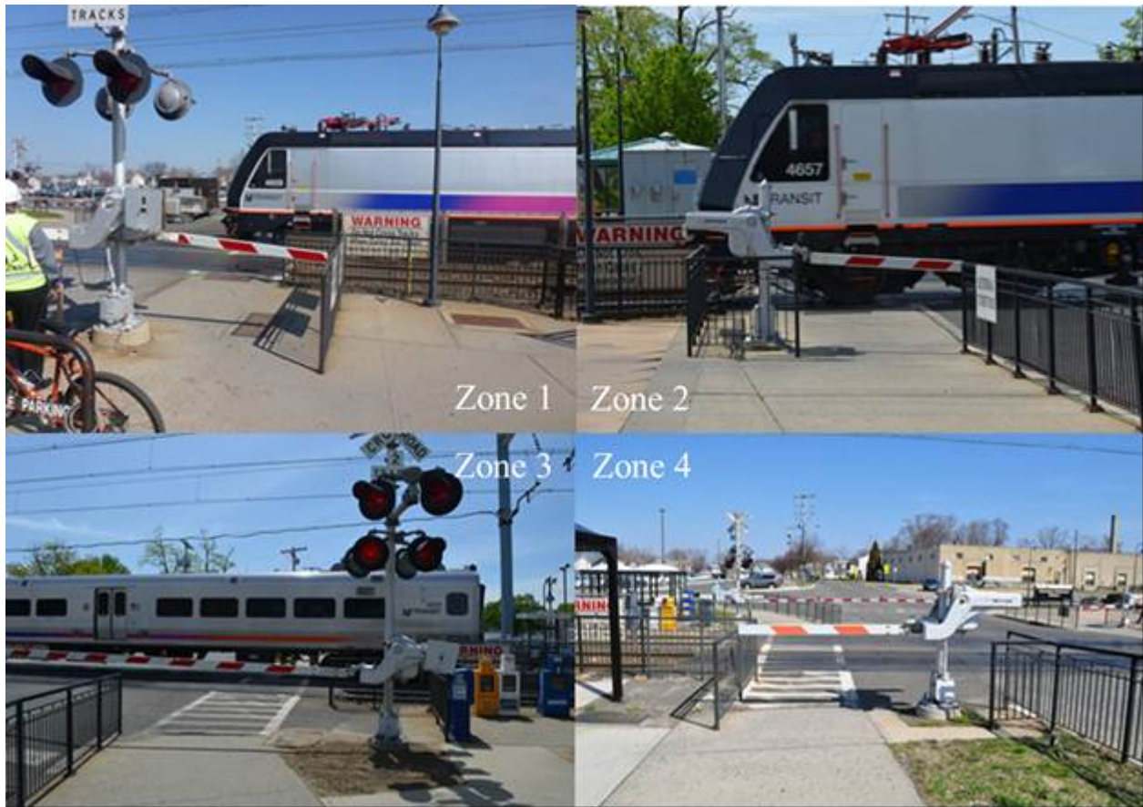
Figure 2. All Four Pedestrian Gates at the Atlantic Ave. Crossing before Installation of Gate Skirts
