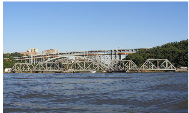
Exhibit 2-2 - Spuyten Duyvil Bridge over Harlem River
