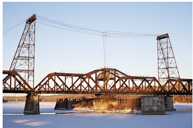
Exhibit 1-3—Livingston Avenue Bridge
