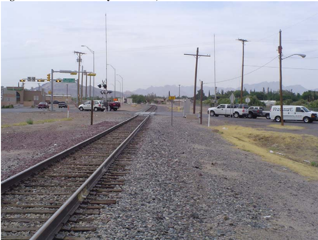
Figure 2F. – BNSF railway in El Paso, Texas
