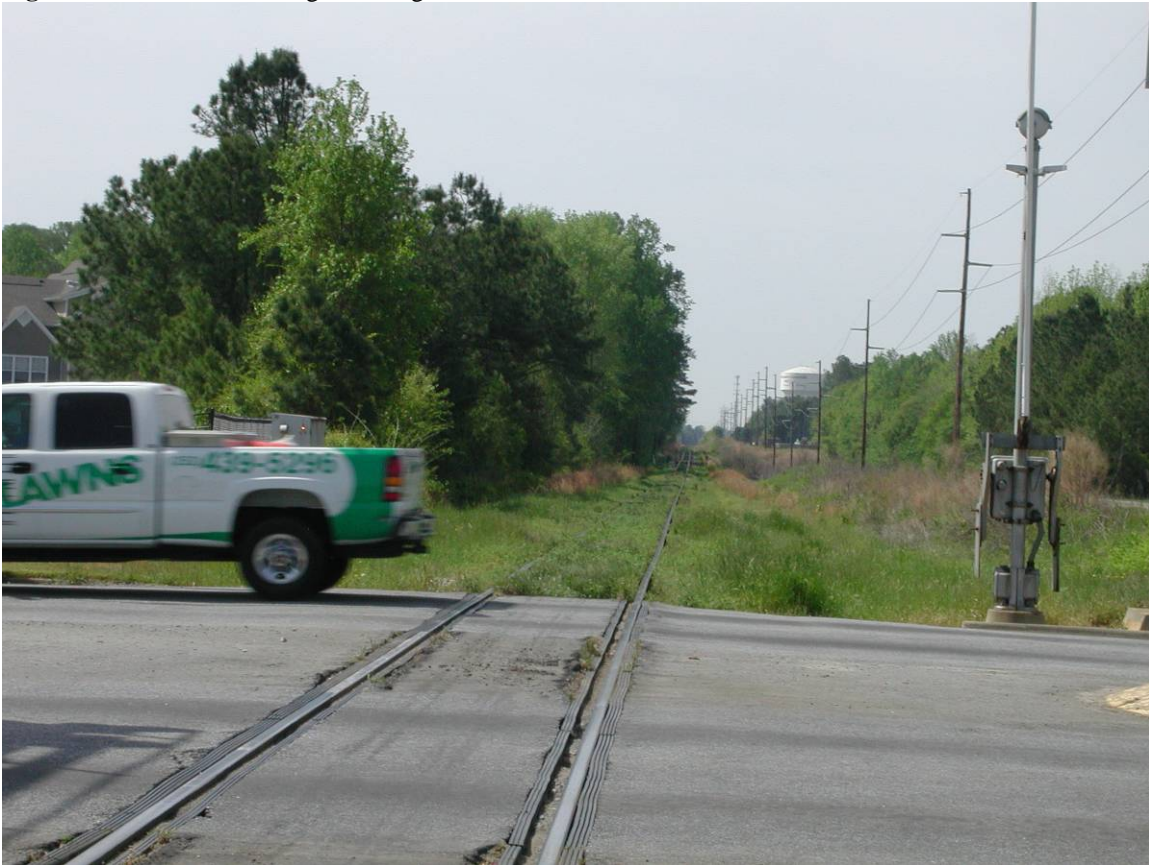
Figure 3.- At Grade Crossing of Arlington Boulevard & CSX railroad
