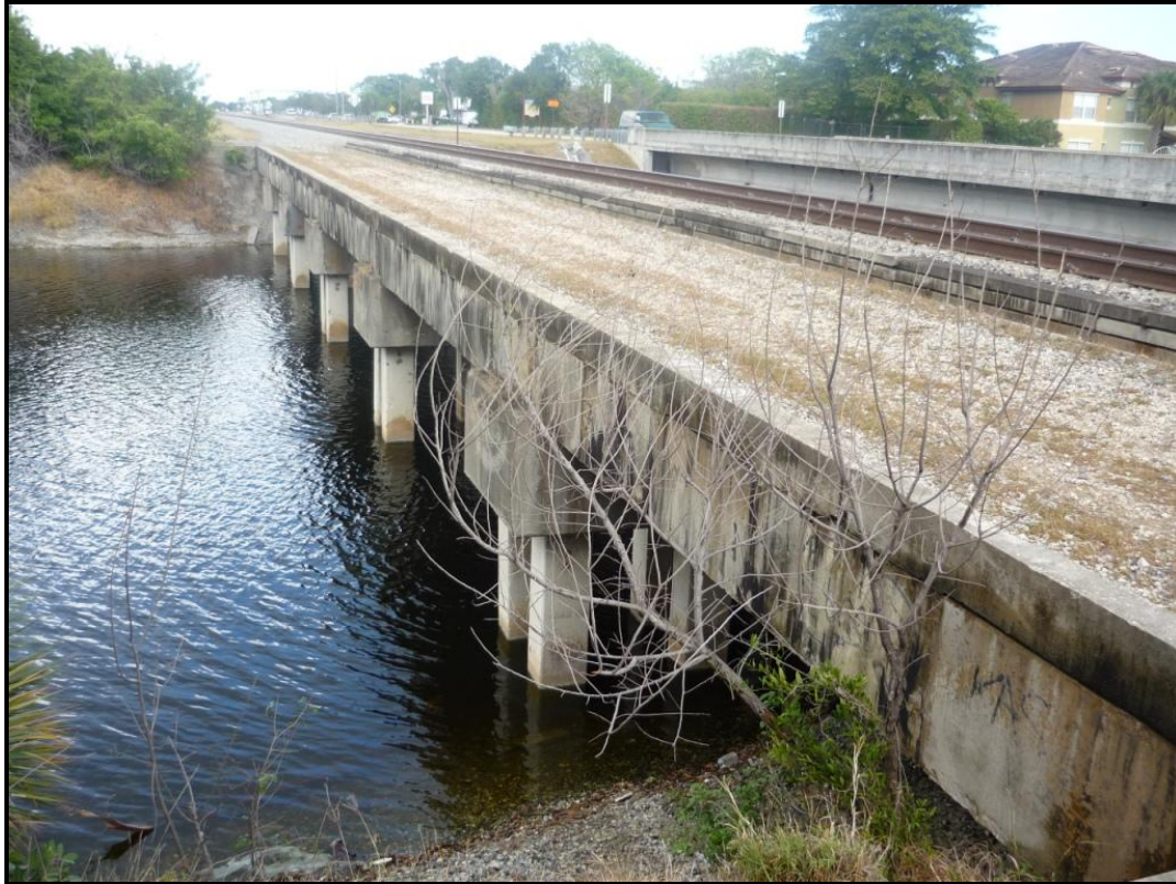
Figure 3. Typical Track Configuration at Single Track Bridge
