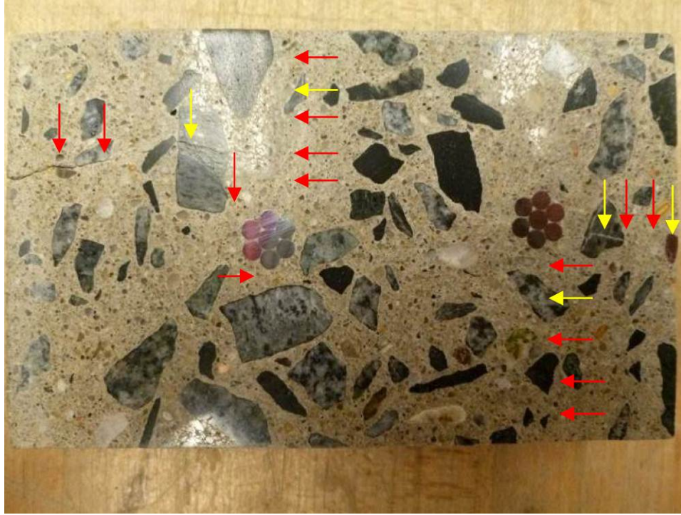
Figure 4.13. Overview of polished section from Core C8-4 showing alignment of cracks.
