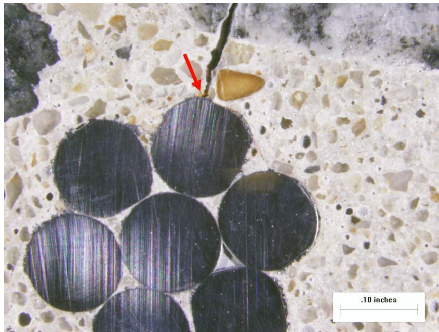
Figure 4.18. A magnified view of the polished cross-section in Core C17-3 at the tendon near the exterior surface. Red arrows point to the minor brown corrosion staining at the tendon.
