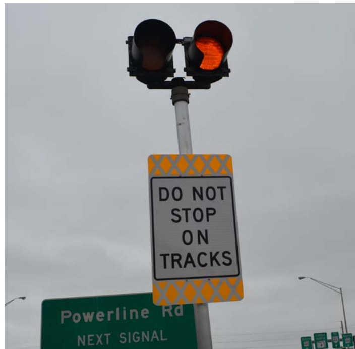
Figure 6. Dynamic Envelope Zone Modified Signage at Commercial Boulevard
