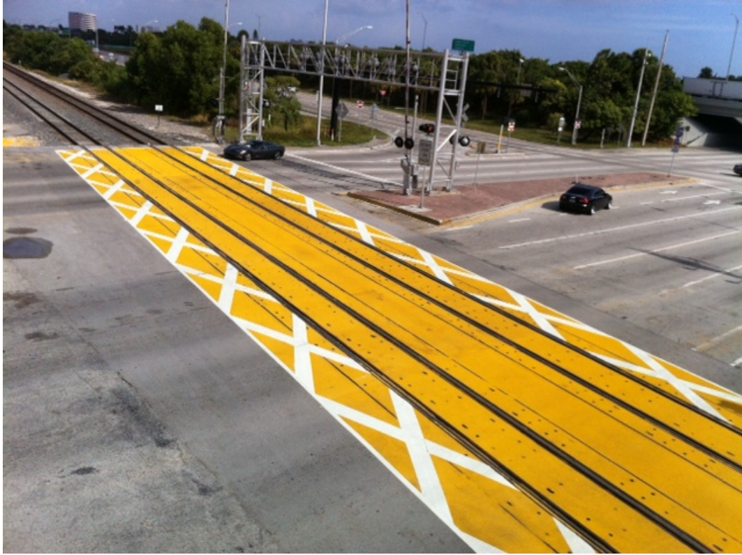
Figure 5. Dynamic Envelope Zone Pavement Markings at Commercial Boulevard
