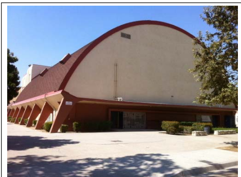
Photo No. 6. View west toward girl's gym (Photograph taken on 9/28/2011).
