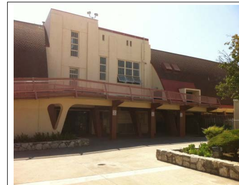
Photo No. 7. View southwest toward north elevation of center section of gym (Photograph taken on 9/28/2011).
