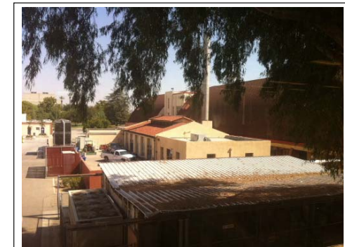
Photo No. 8. View east toward Boiler Room with red tiled roof (Photograph taken on 9/28/2011).
