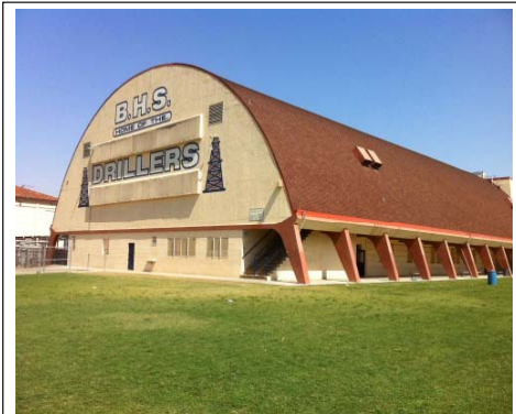
Photo No. 5. View northeast toward west end of Gymnasium (Photograph taken on 9/28/2011).
