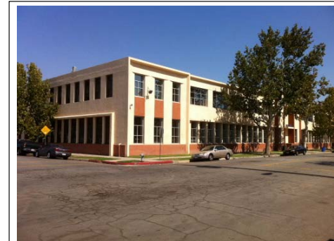
Photo No. 11. View northeast toward west elevation and facade Of 1920s Industrial Arts building (Photograph taken on 9/28/2011).
