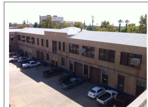
Photo No. 12. View southeast toward north elevation Of 1920s Industrial Arts building (Photograph taken on 9/28/2011).
