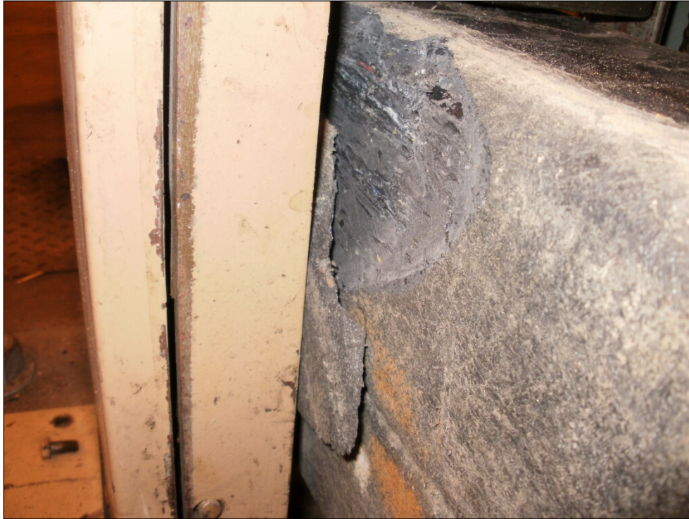
Figure 31. Surface damage (large chip) on tie after drop test, room temperature.
