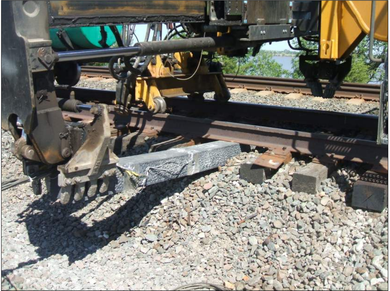
Figure 19. Instrumented tie during insertion at the BNSF site.
