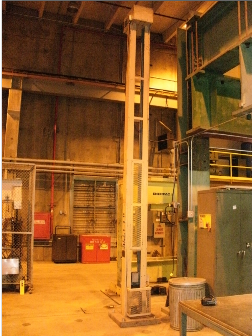
Figure 28. Drop load fixture located at TTC in the Component Test Laboratory.
