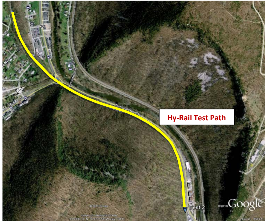
Figure 8: Hy-Rail LIDAR testing was performed along a section of the Western Maryland Scenic Railroad (highlighted in blue)
