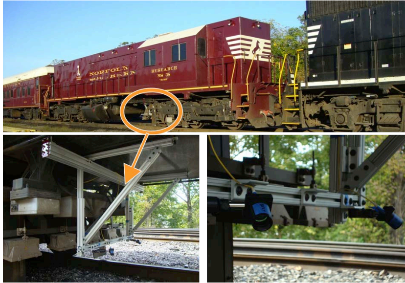
Figure 22: LIDAR system installation onboard the rail geometry car
