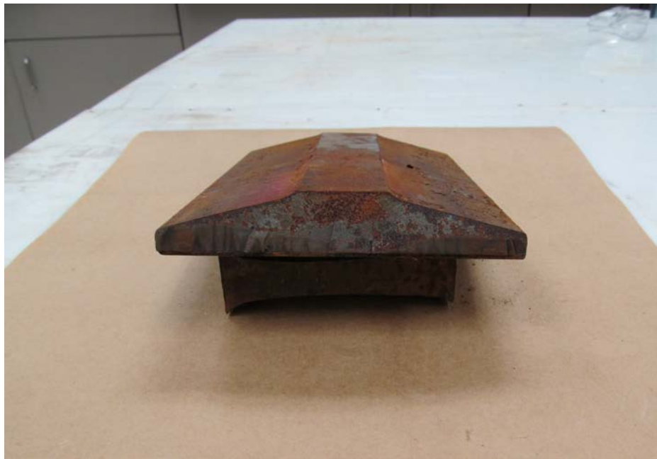
Figure 37. Fracture Surface of Corroded Sample with ALL Treatment
