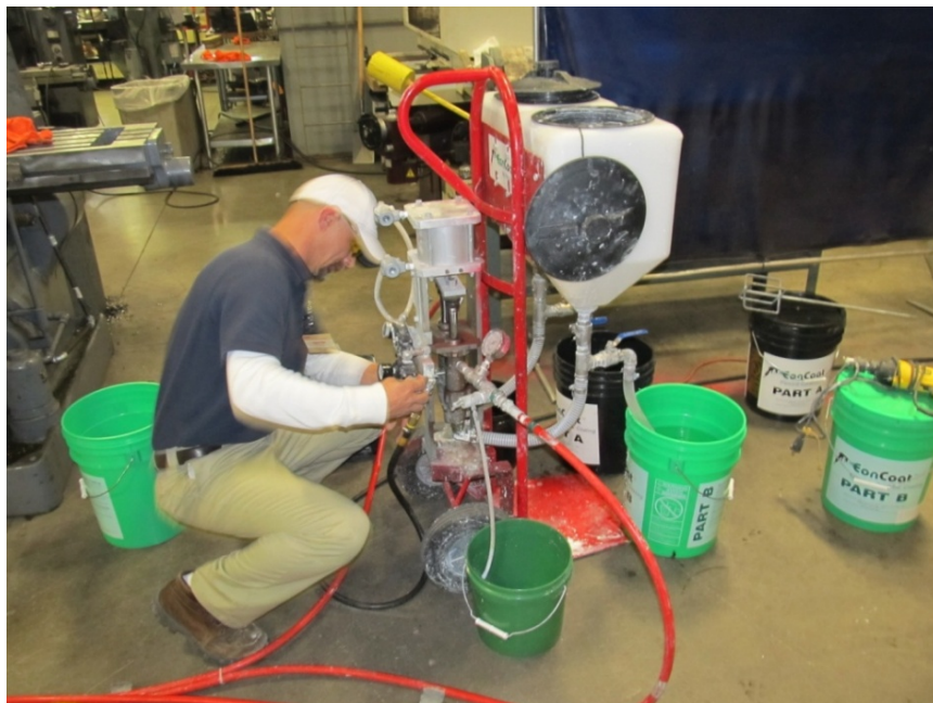
Figure 14. Technician Readies EonCoat® Applicator System
