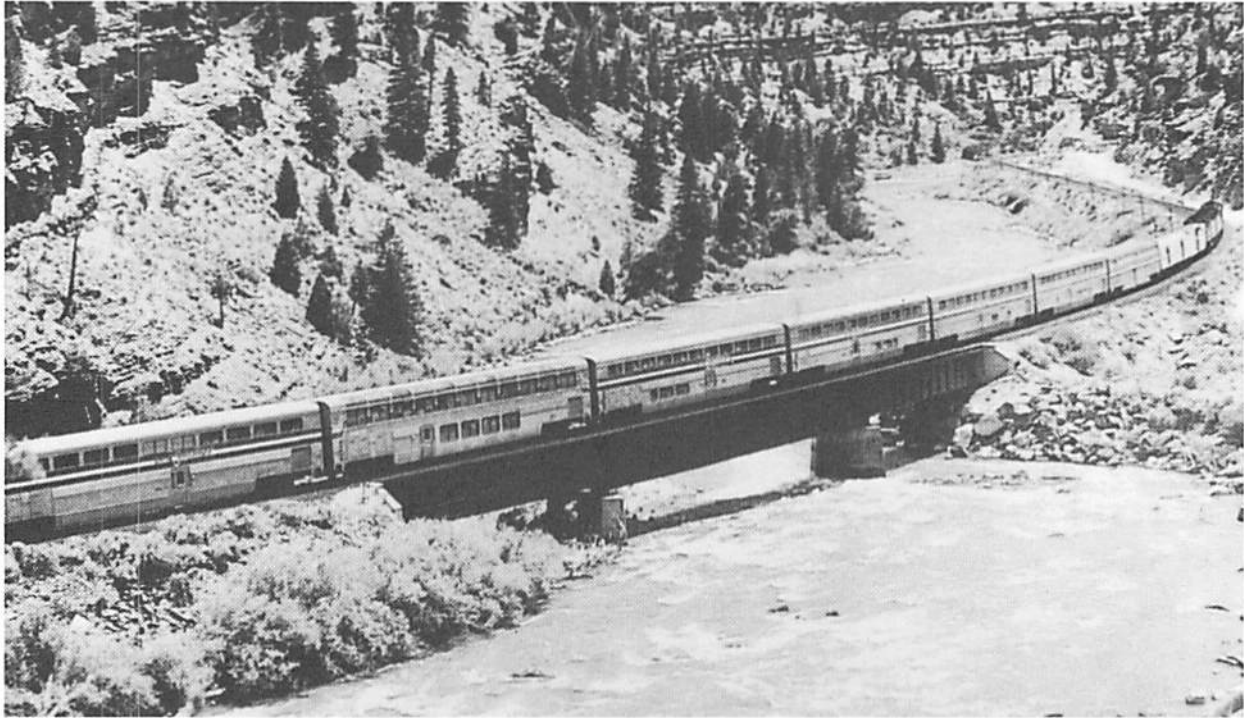
Figure 2-9. Intercity Passenger Train Operating Over a Bridge
