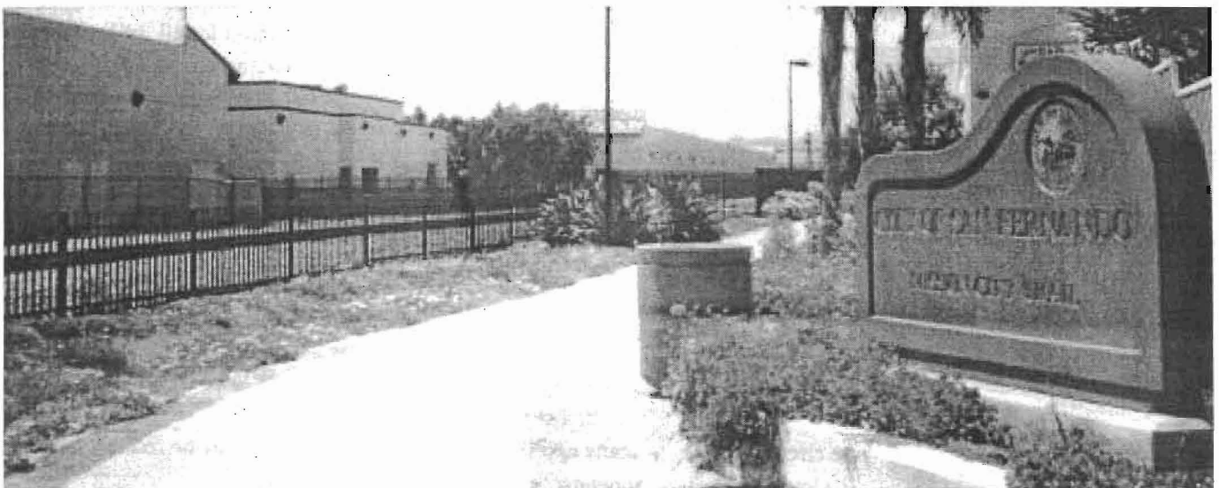
Wrought iron fencing offers an aesthetically-pleasing option. Mission City Rail Trail, San Fernando, CA
