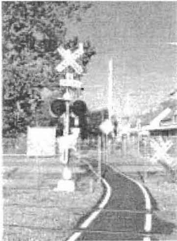
Dual track grade crossing. Burlington, VT
