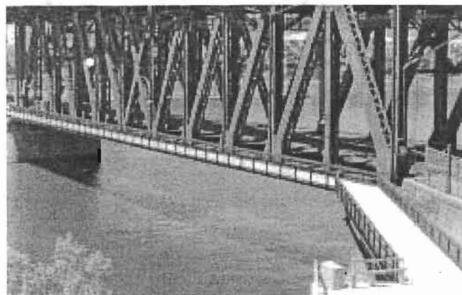
Narrower setback distances may be acceptable, as on this Union Pacific railroad bridge with slow-moving trains. Steel Bridge Riverwalk. Portland, OR
