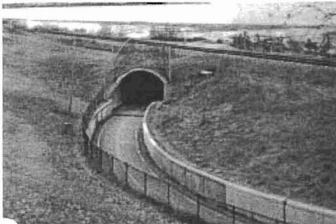
Undercrossing of Alaska Railroad Corporation tracks, Tony Knowles Coastal Trail. Anchorage, AK
