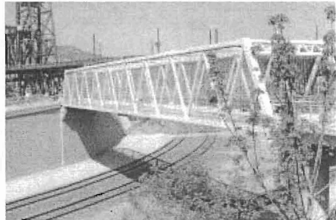
Overcrossing of Union Pacific tracks. Portland, OR
