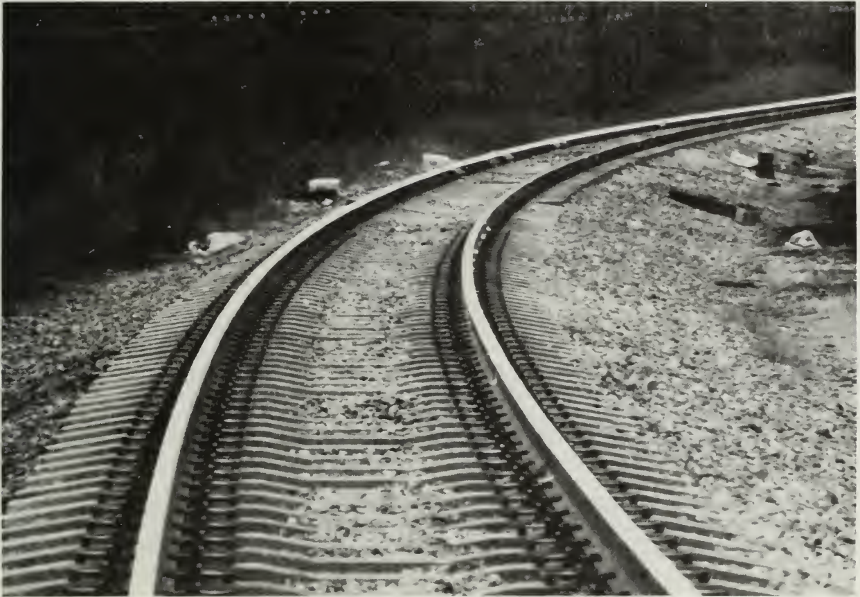
FIGURE 6. CHESIE CONCRETE TIE TEST TRACK, RICHMOND (LORRAINE), VA., (3 DEGREE CURVE)
