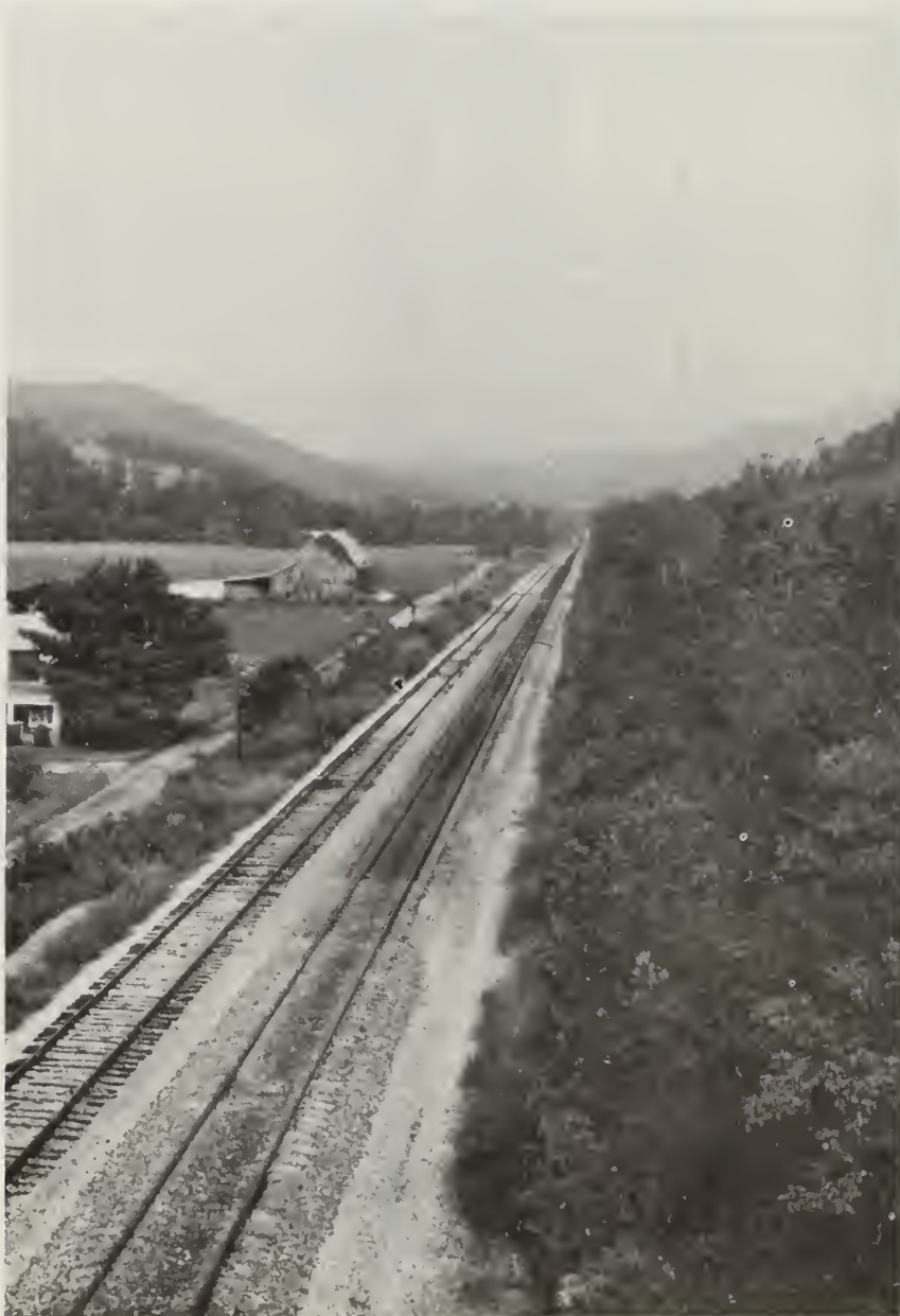
FIGURE 11. N&W CONCRETE TIE TEST SITE, NEAR ROANOKE, VA., LOOKING WEST
