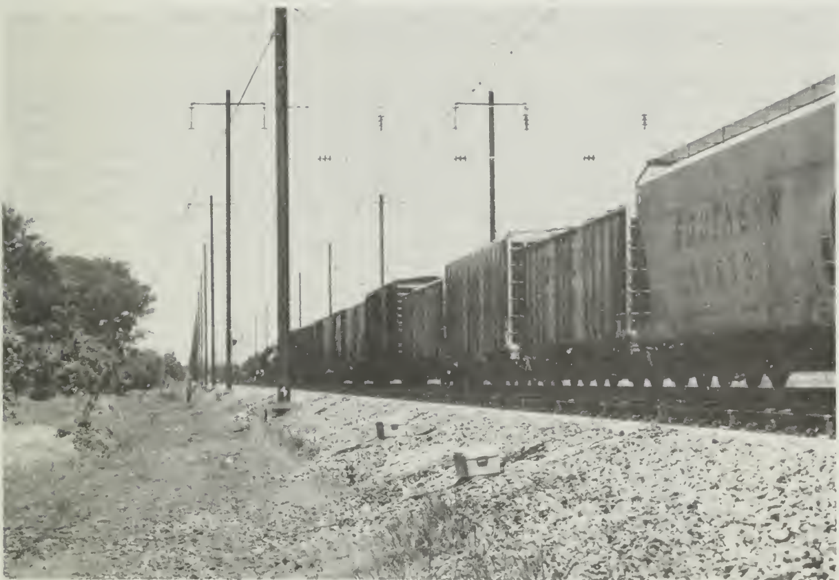
FIGURE 9. VIEW OF ABERDEEN TEST SITE LOOKING NORTHEAST
