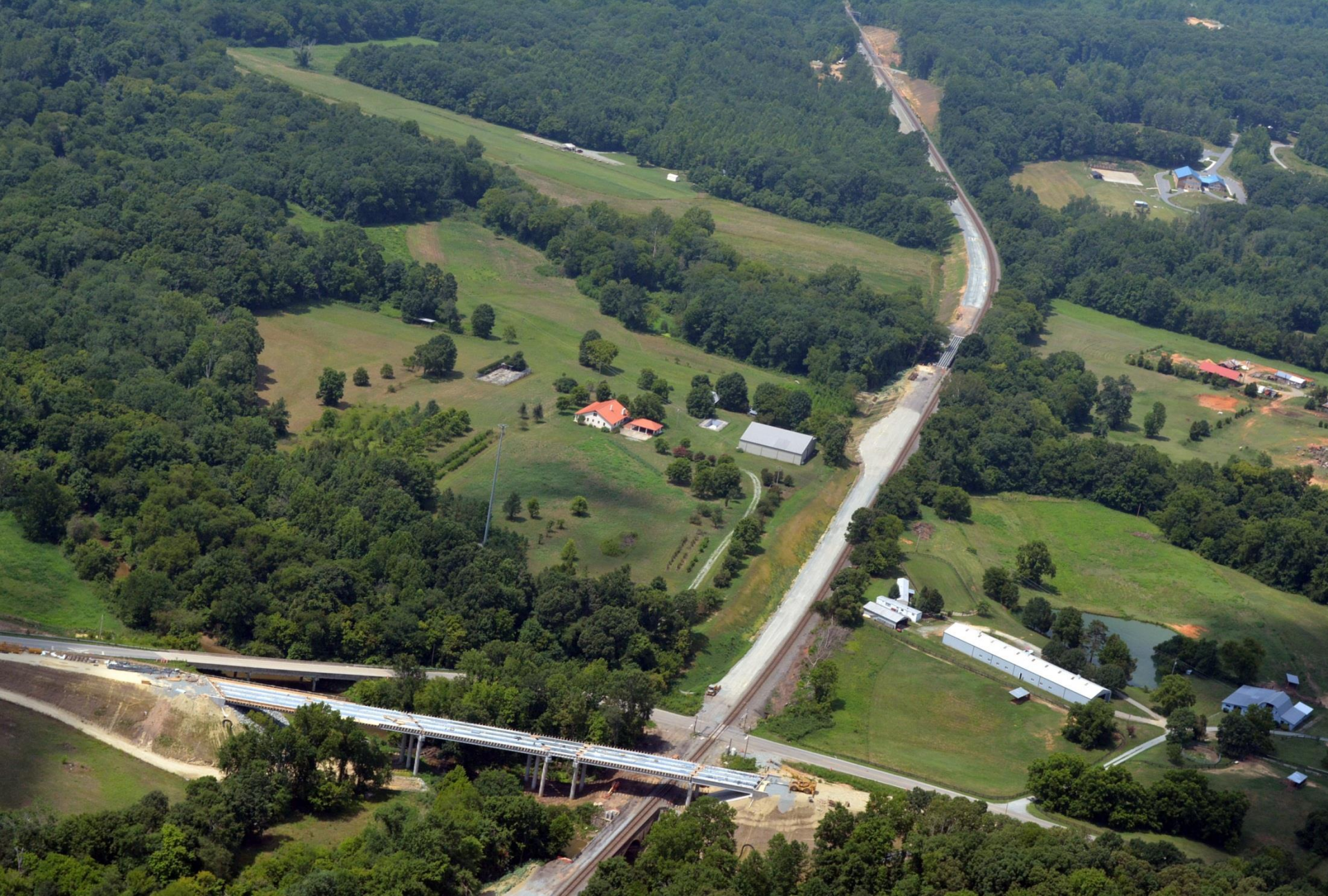
Bowers to Lake Double Track Project: Turner Road Grade Separation
