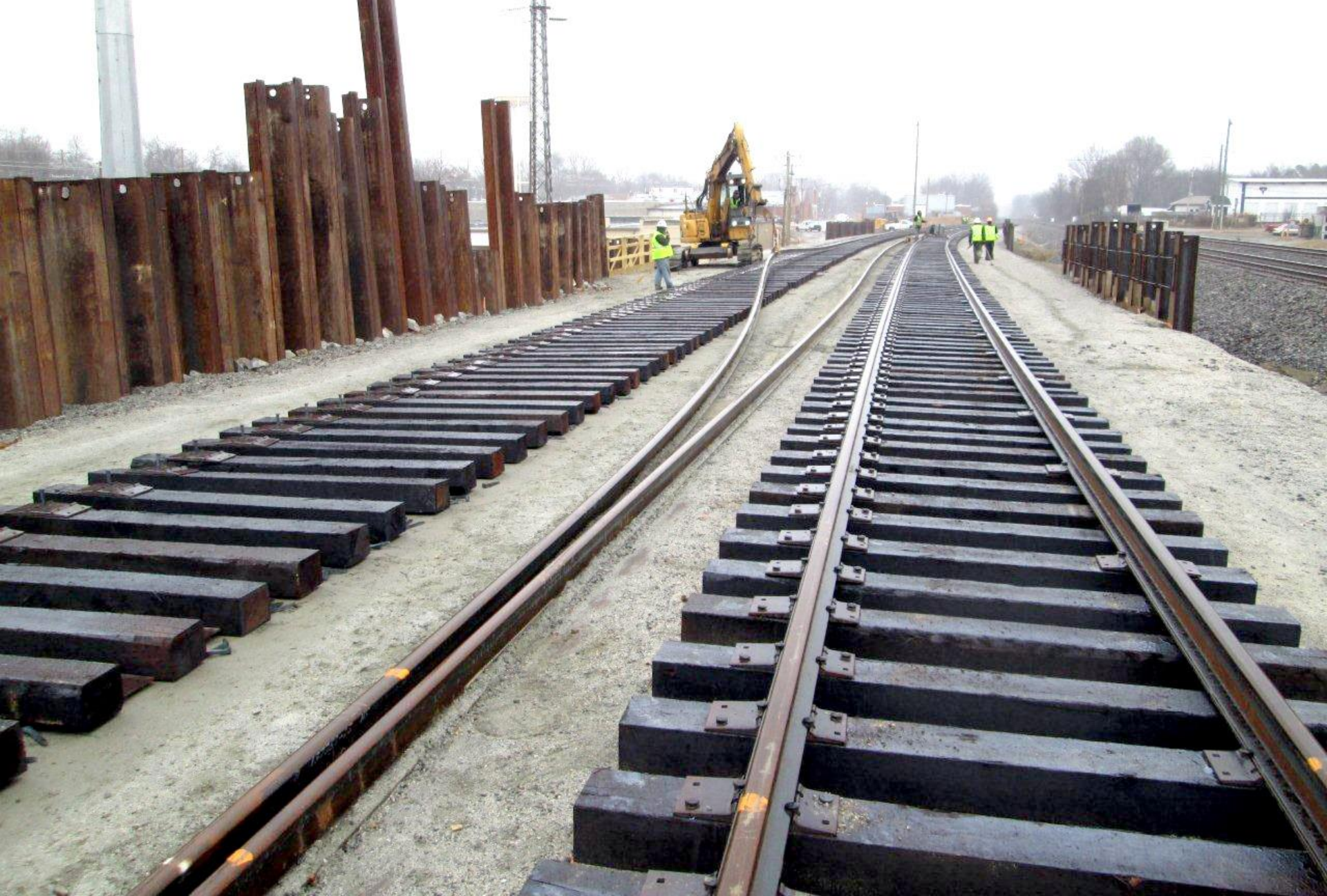
Klumac Road Grade Separation: Bypass Track
