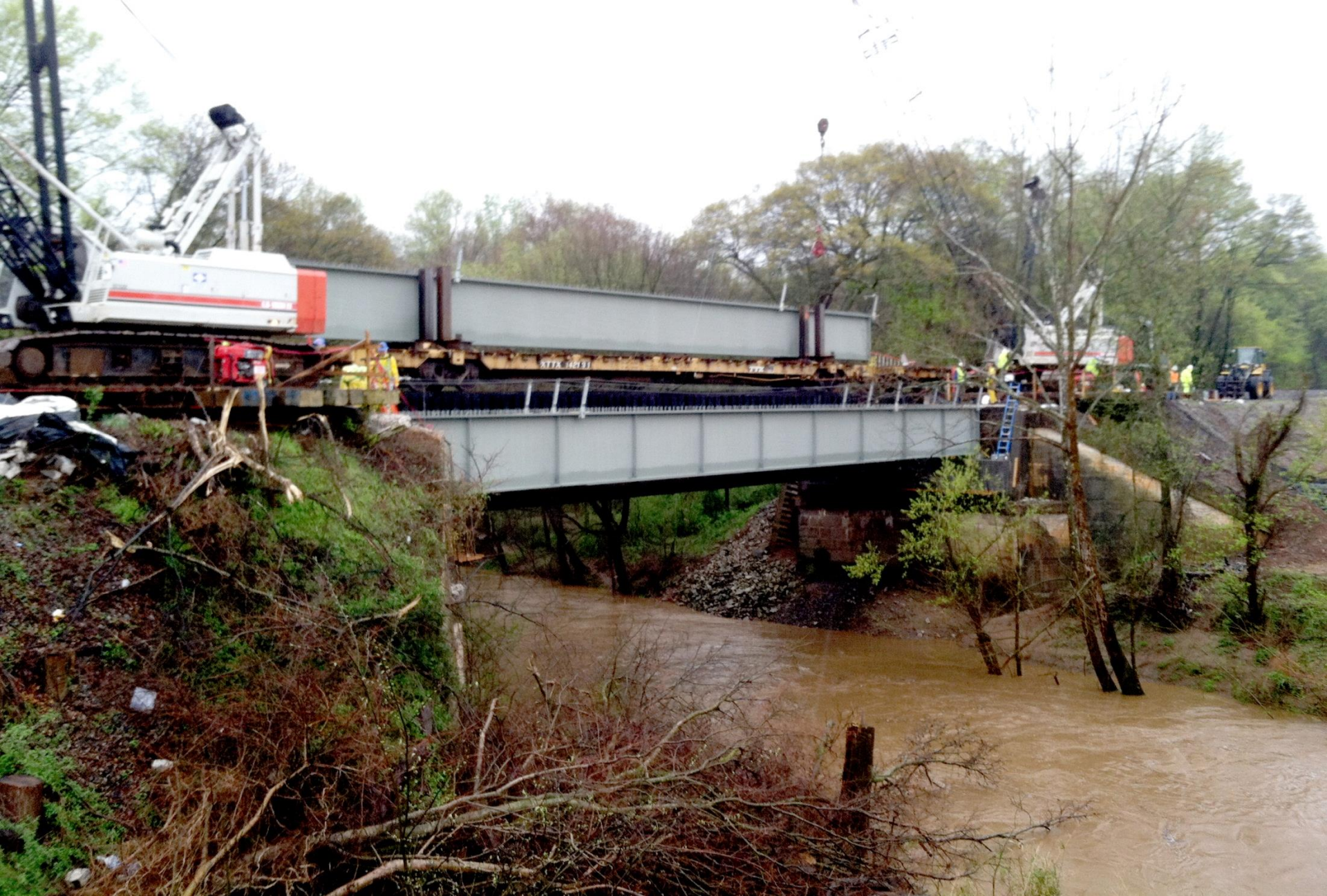
Haydock to Junker Double Track Project: Rocky River Bridge
