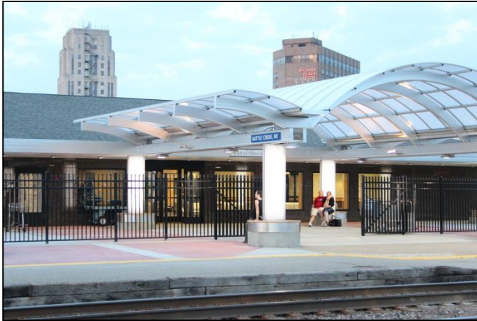
Battle Creek Station - Renovation
