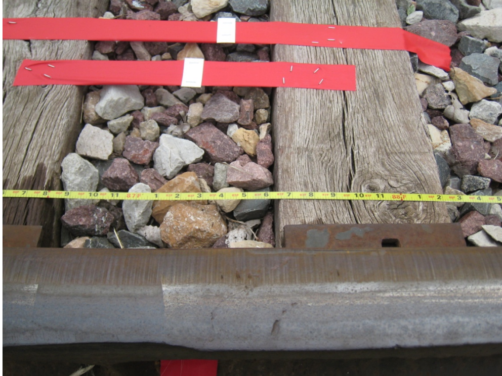
Figure 10.2. Reflective Targets Placed in Correspondence of Joints, Weld, and Defects
