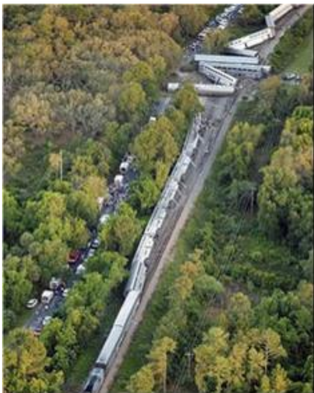
Figure A4. Aerial View of Crescent City Derailment on April 18, 2002 (from NTSB report)
