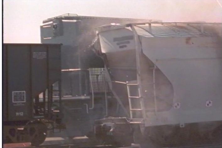
Figure 14. Locomotive Right Rear Contacts Damaged Covered Hopper Car
