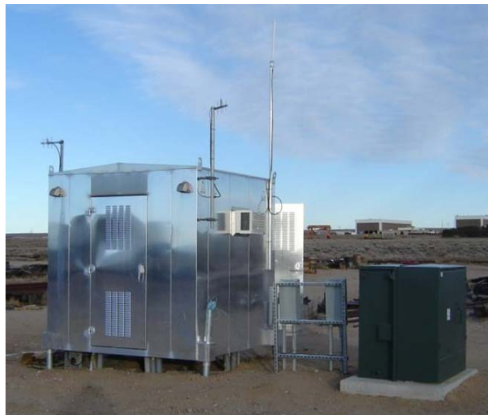
Figure 15. 602 Bungalow at RTT Siding Turnout
